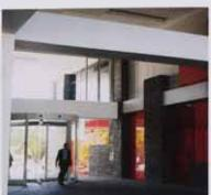
Facing page: A concrete blade follows the line of the northwestern section of the building in a square arch. This bold visual statement has a practical purpose in that it shades the plant room where the building's systems are housed.
